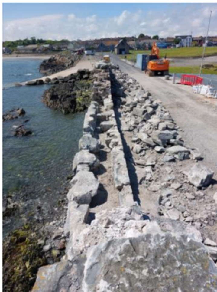
Core between inner and outer skins filled to remove voids
