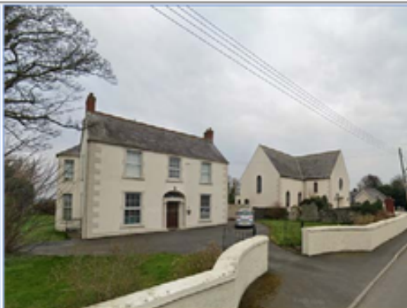
Figure 11 - Manse and Listed Church Opposite Site
