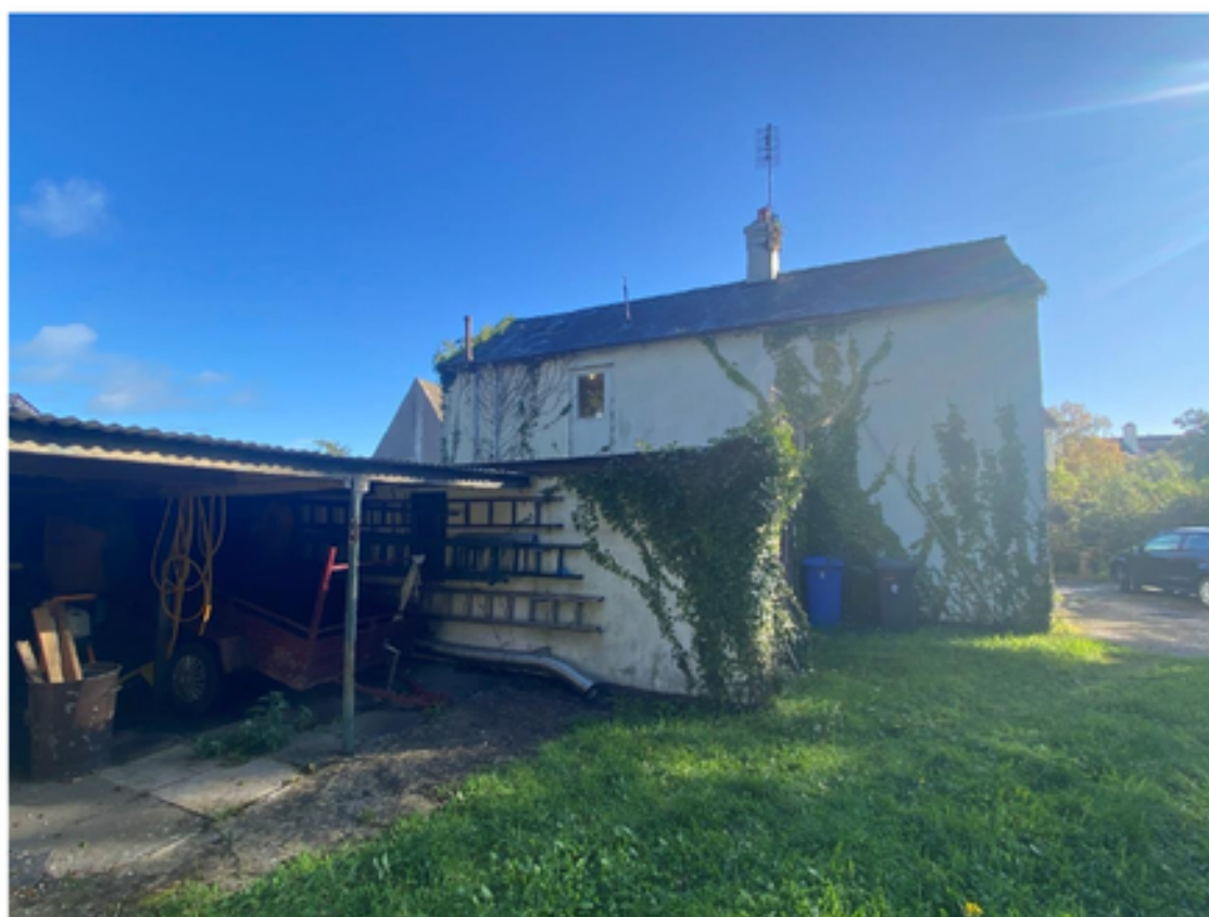
Rear Elevation of existing dwelling (west)
