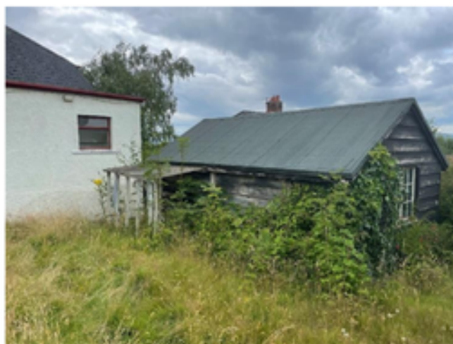
Figure 3 - Garage proposed to be demolished.
