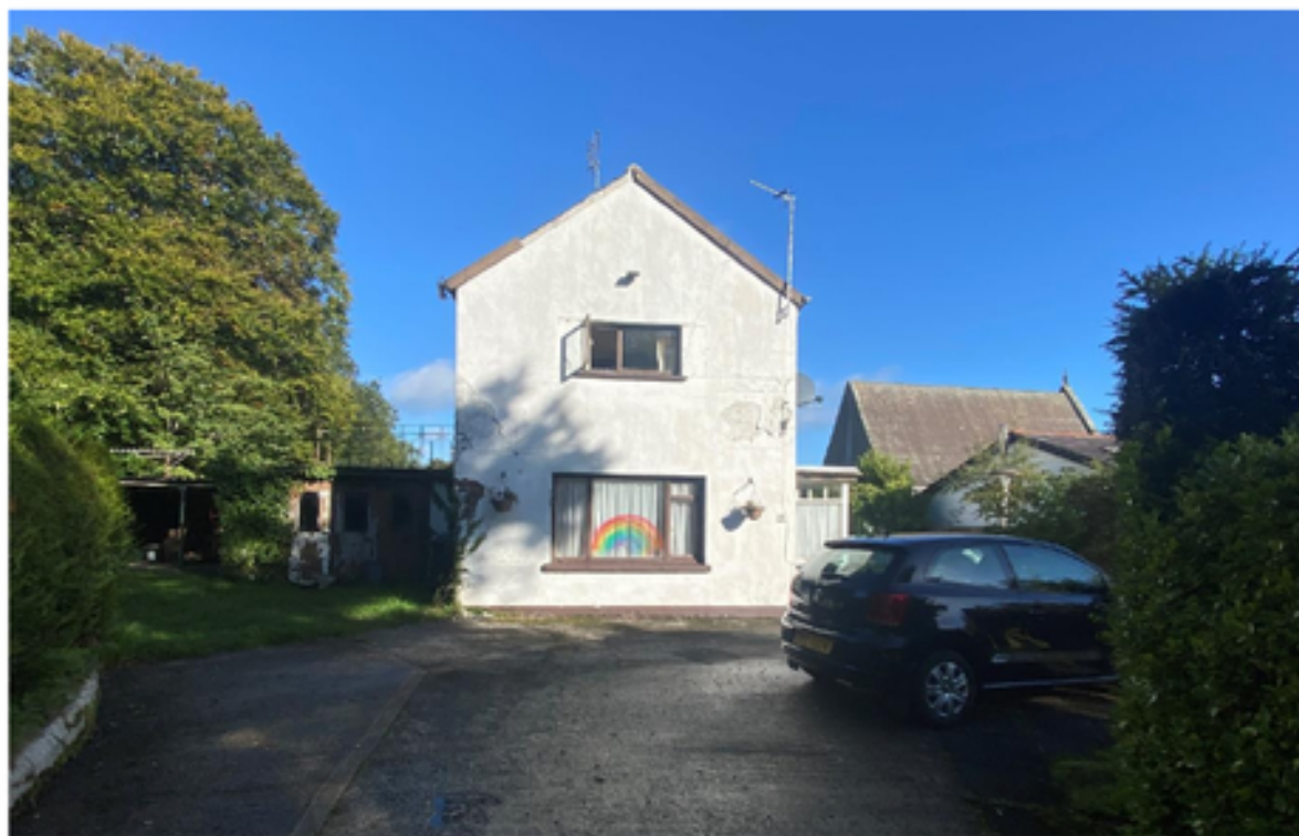
Gable elevation of existing dwelling – on approach from driveway
