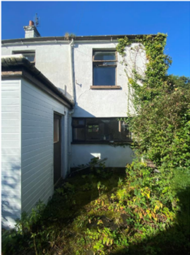
Images showing existing condition of dwelling
