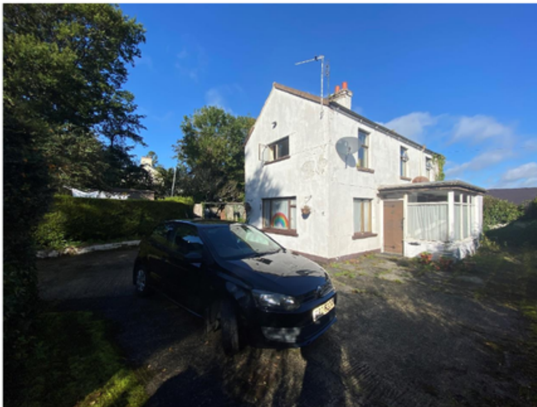
Front Elevation of existing dwelling with small single-storey porch to front
