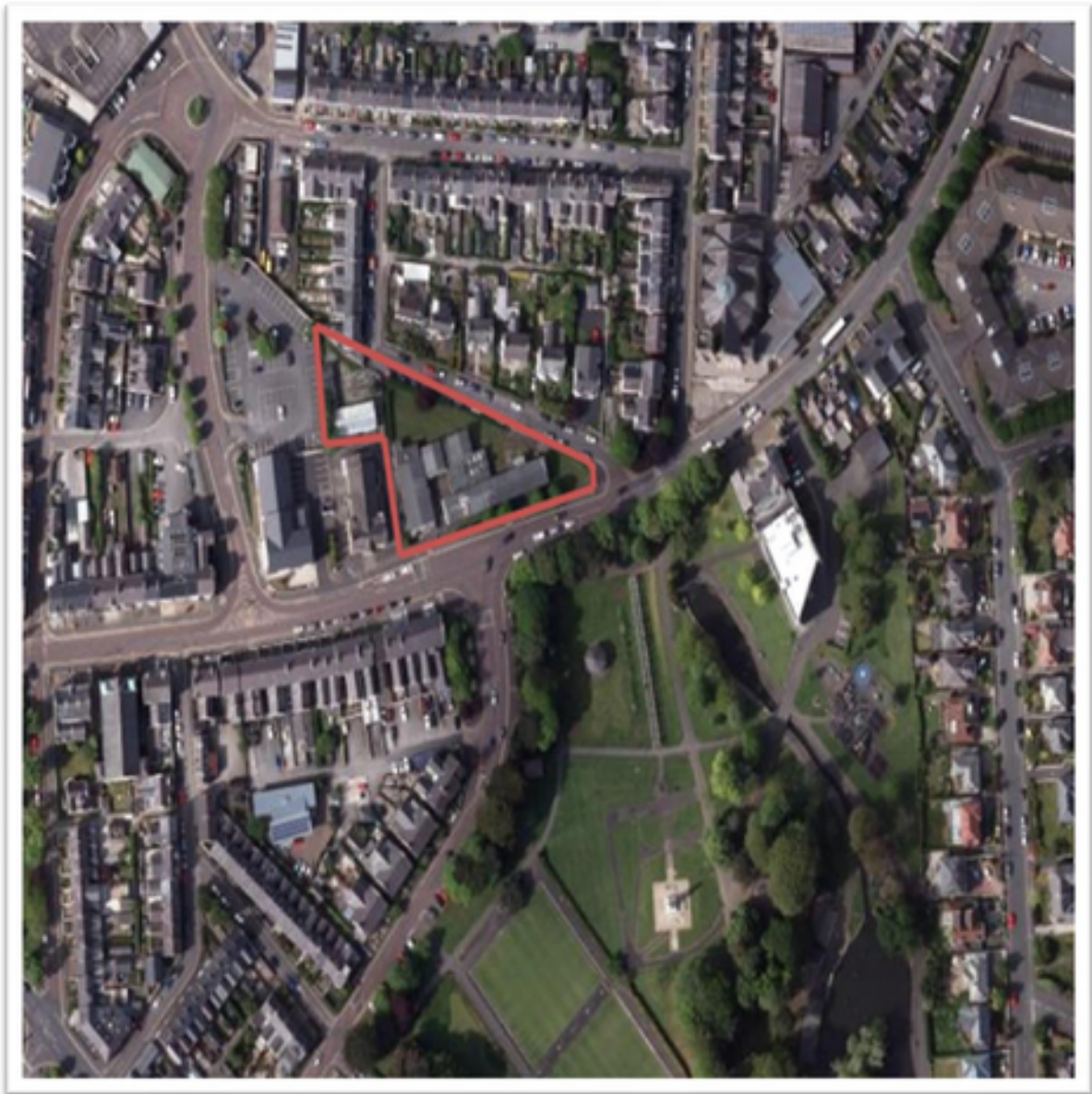
Aerial view of site outlined in red and showing footprint of former buildings now demolished
