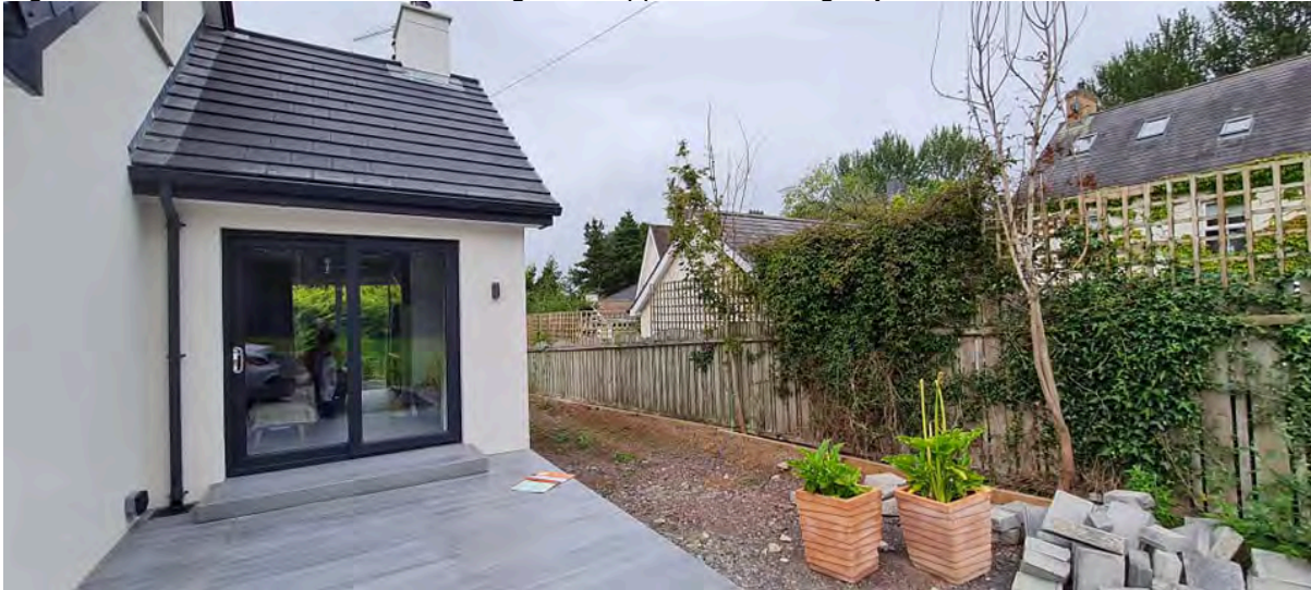
Figure 8: Patio area of No 1A The Grange with applicant building adjacent
