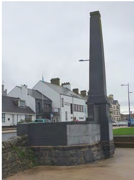
Viewed from coastal side
