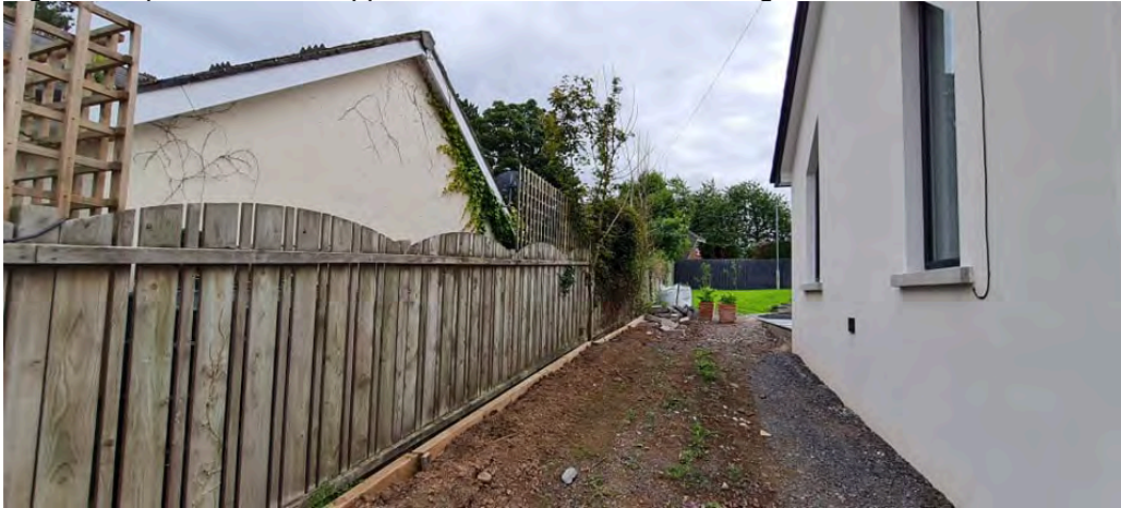
Figure 6: Space between application site and 1A The Grange
