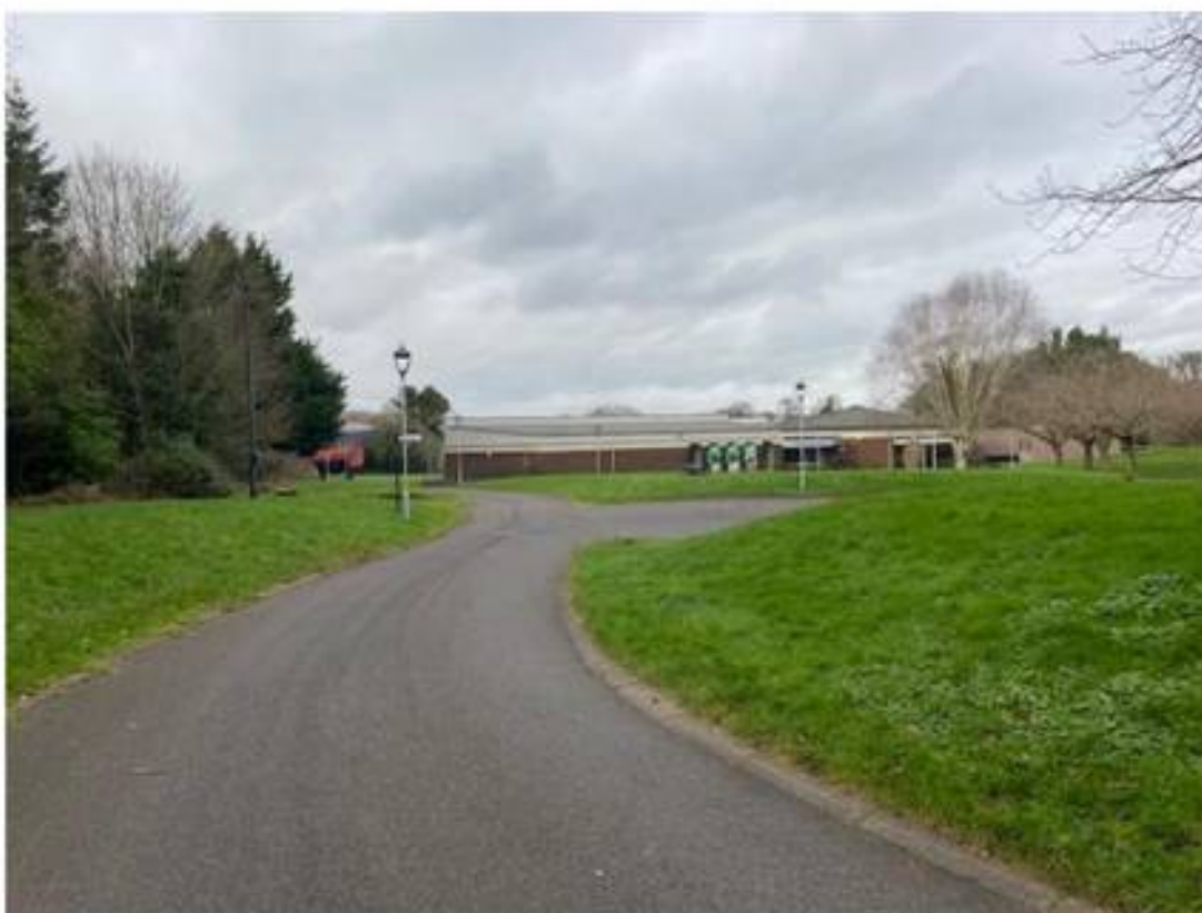
Existing road and museum building located at southern end of the site
