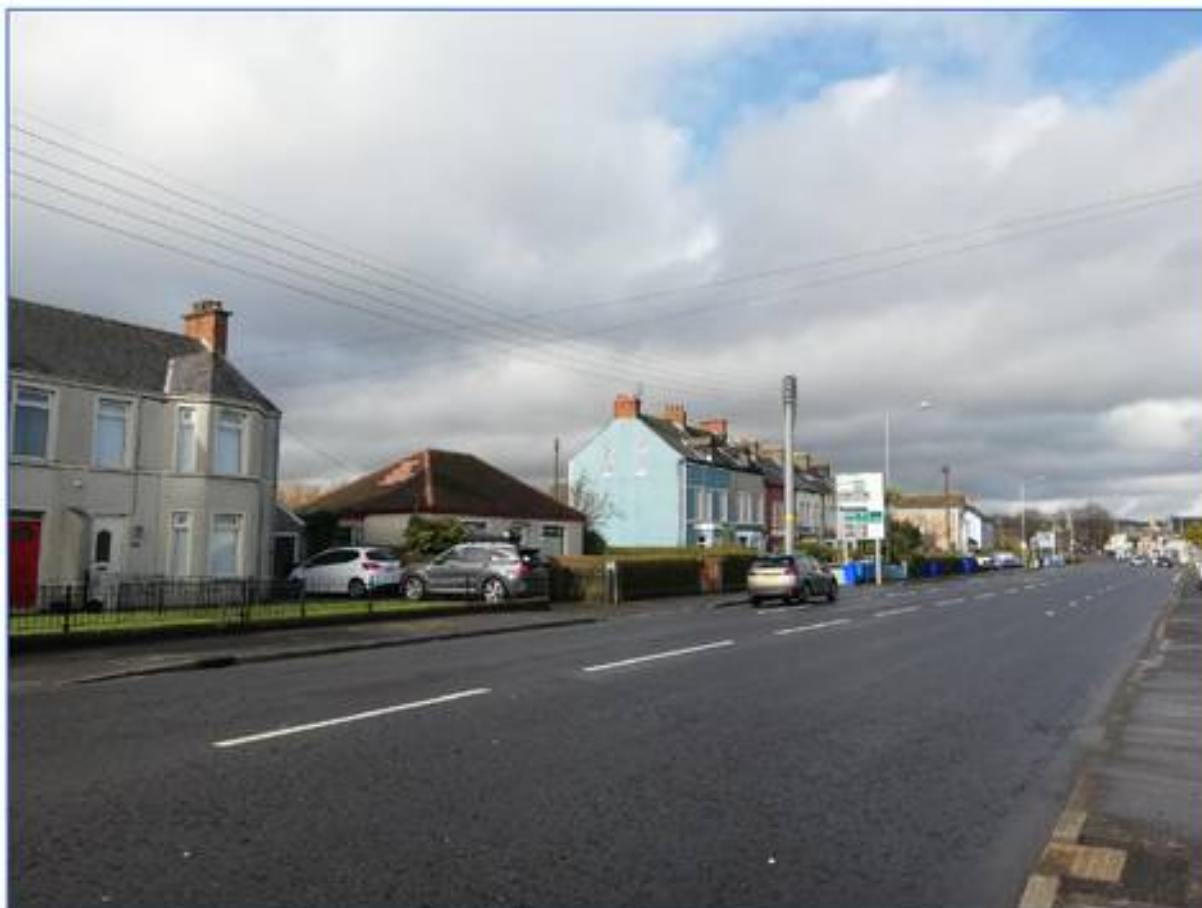
Figure 7 – Existing Properties Along Portaferry Road
