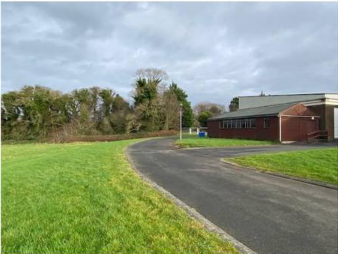
Road curves at southern end of site to meet up with new path that will lead to coastal path
