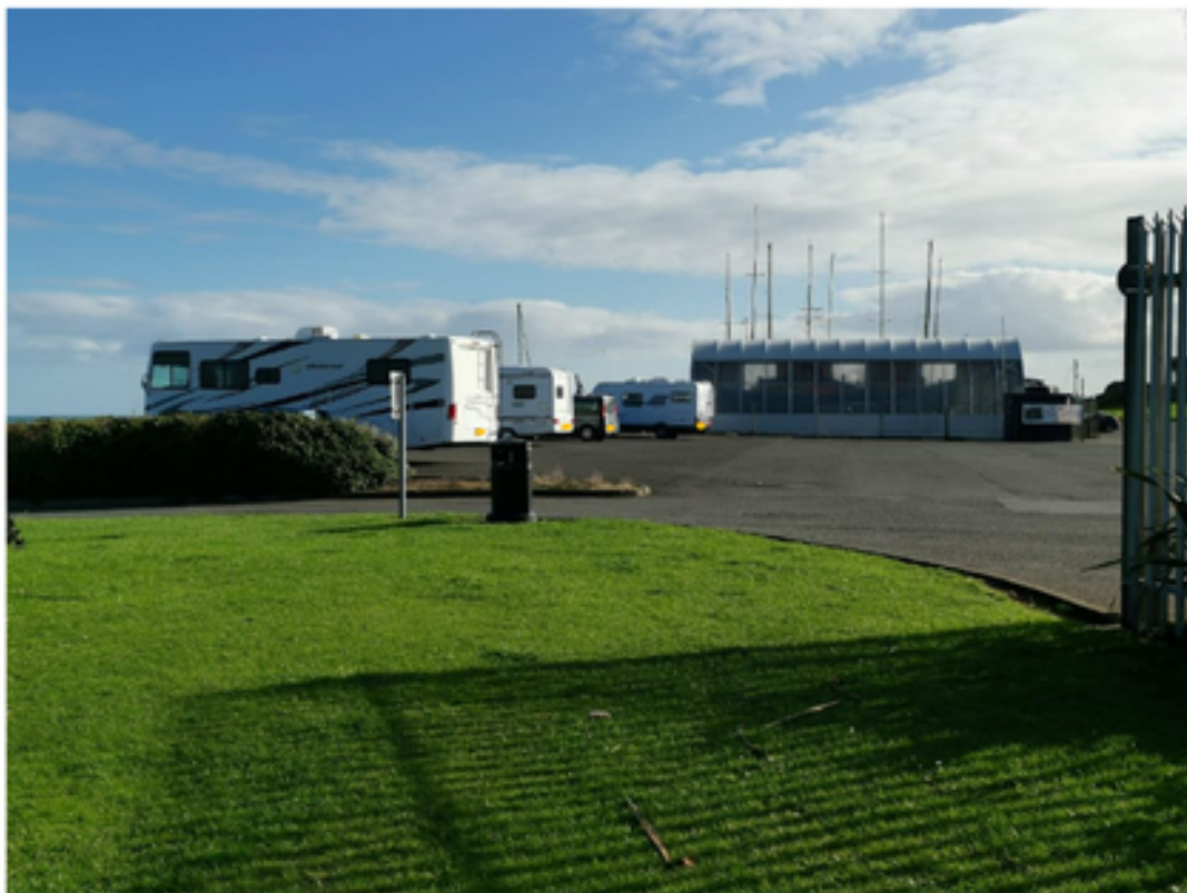
Photo 14 Sir Samuel Kelly Lifeboat & Shelter, Donaghadee Car park view near entrance
