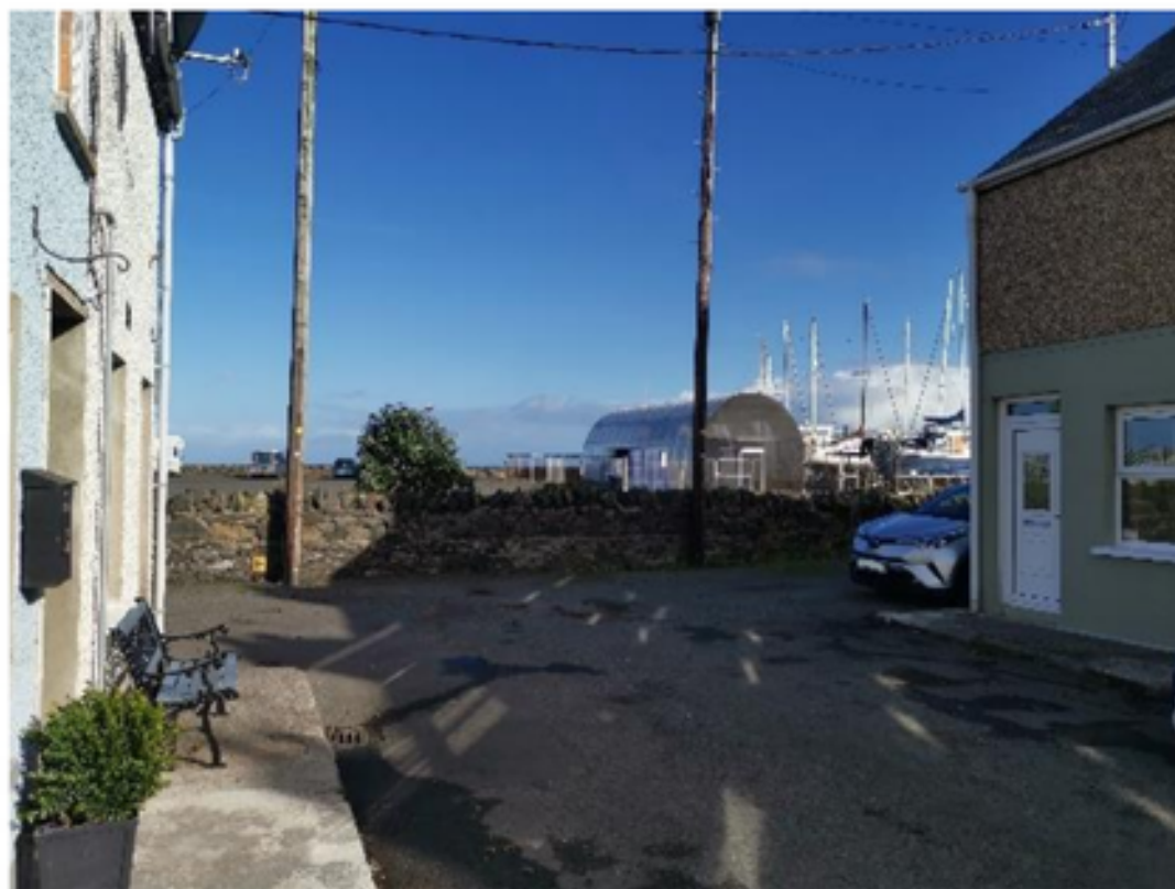
Sir Samuel Kelly Lifeboat & Shelter, Donaghadee Photo 13 – Neighbouring properties (view from Edward Street)
