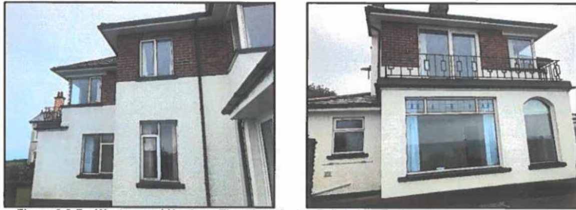
Figure 6 & 7 – Western and Northern Elevations facing Ballyholme Esplanade
