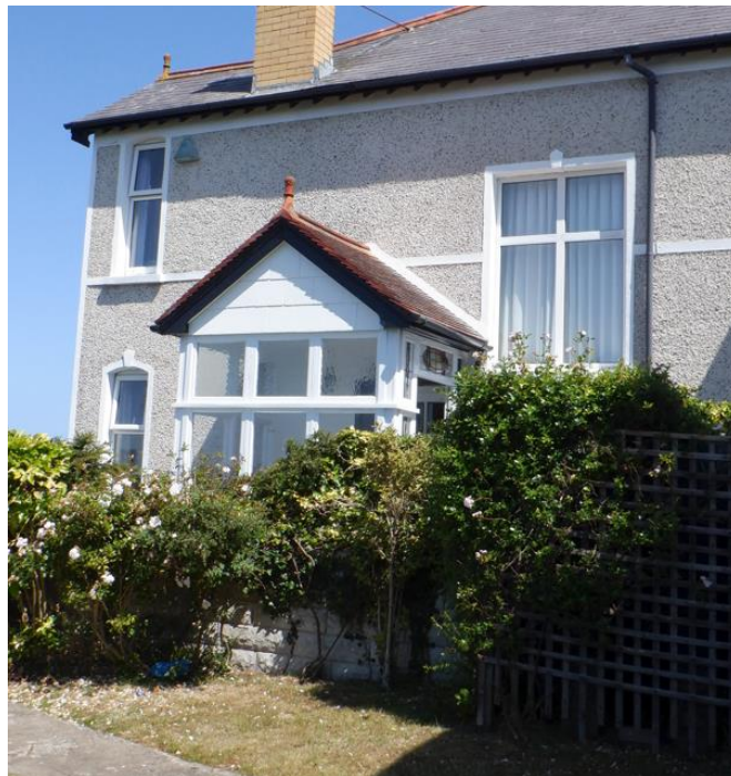
Figure 28 – western side of No.17
