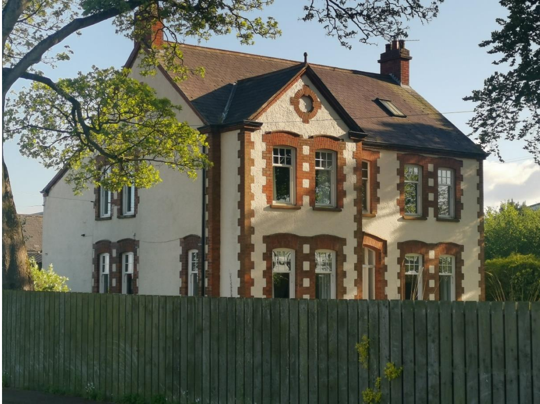
129 Newtownards Road, Comber Photo 5 – View of main house
