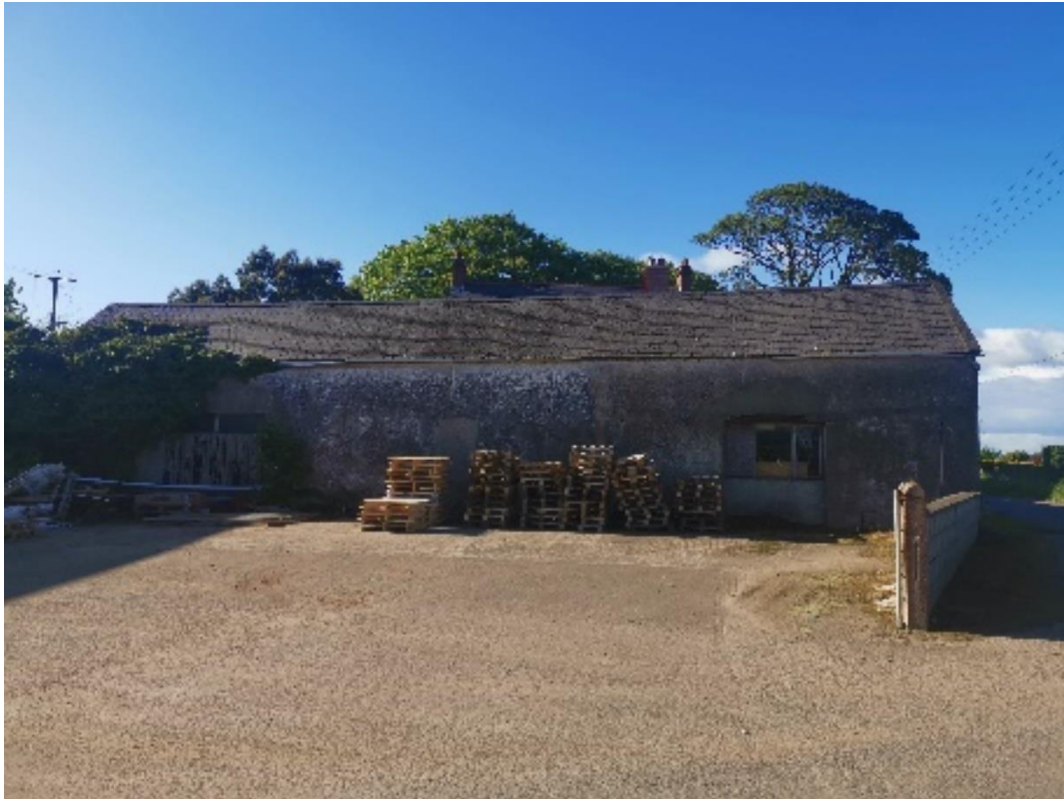
129 Newtownards Road, Comber Photo 11 – Barn adjoining neighbouring farmyard
