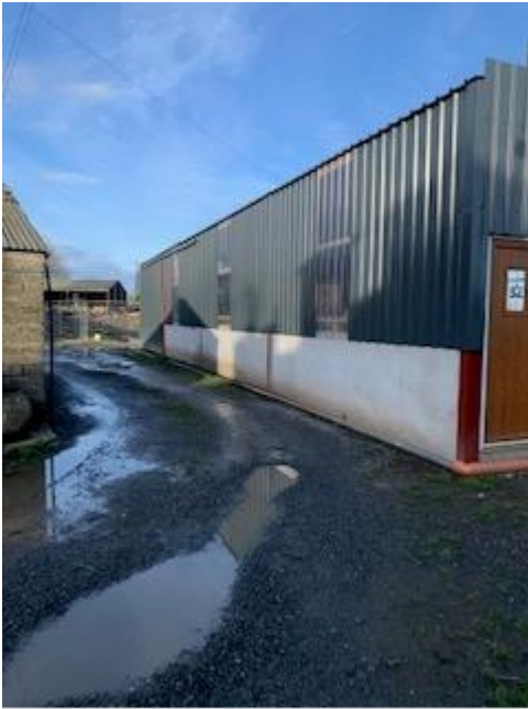
View of retrospective shed
