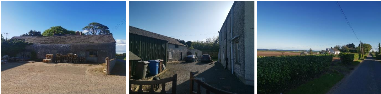
The Barn at 129 Newtownards Road Photos 11, 12 & 13 – Neighbouring Uses & Properties
