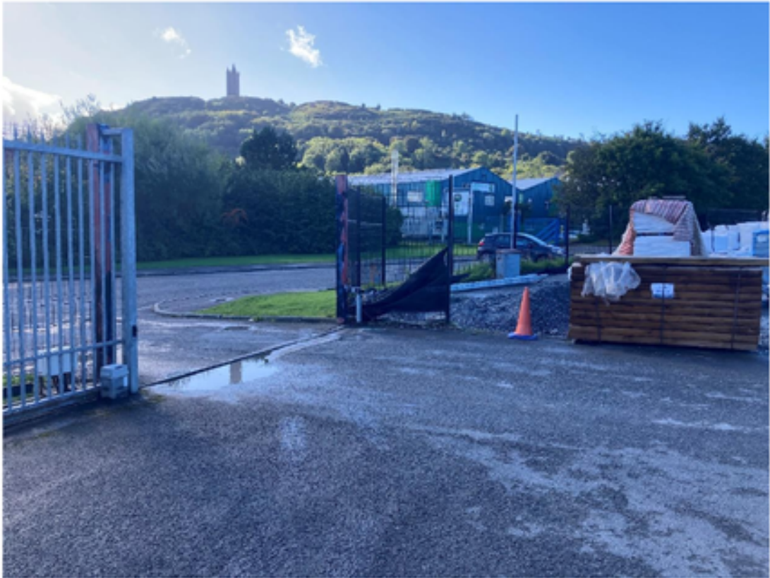
New access in place leading onto Jubilee Road
