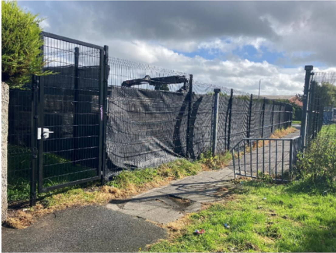
Existing pathway still in place leading from Ardmillan Crescent
