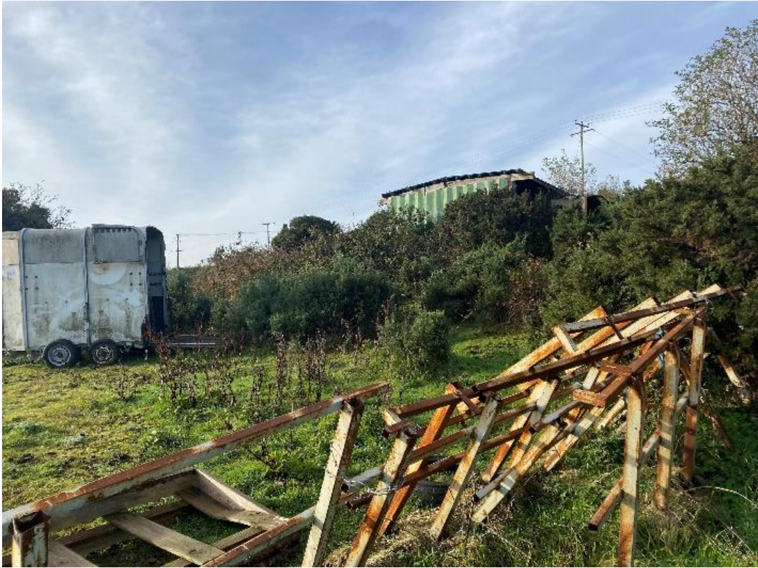
Existing dilapidated shed on site along with scrap metal
