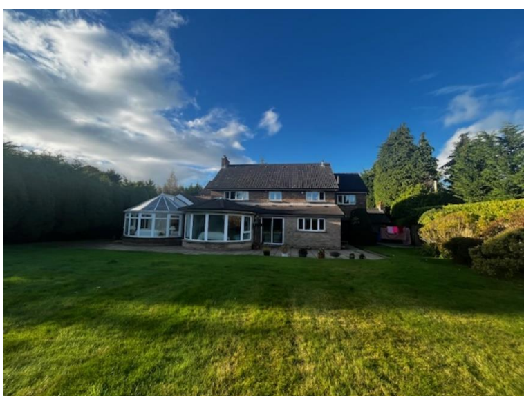
Photo 2: Existing rear elevation, 31 Old Cultra Road.
