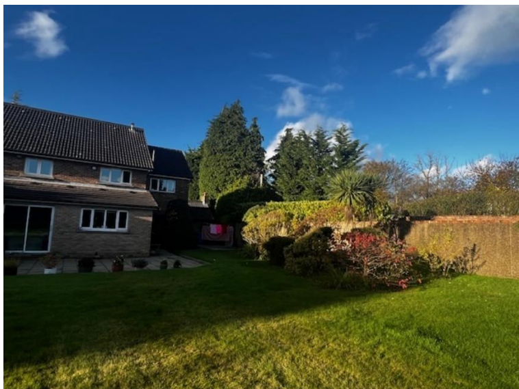
Photo 4: Existing rear elevation of 31 Old Cultra Road.
