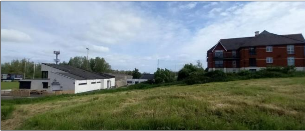
Figure 9: Application Building and Neighbouring Apartments to the Rear
