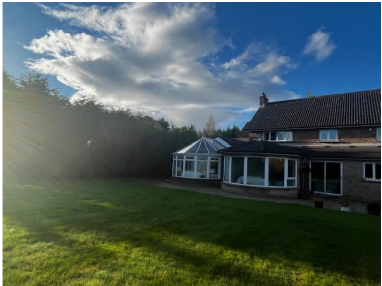
Photo 3: Existing rear elevation of 31 Old Cultra Road.
