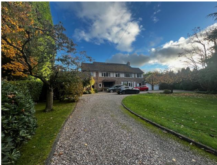
Photo 8: Existing front elevation, garden and driveway, 31 Old Cultra Road.
