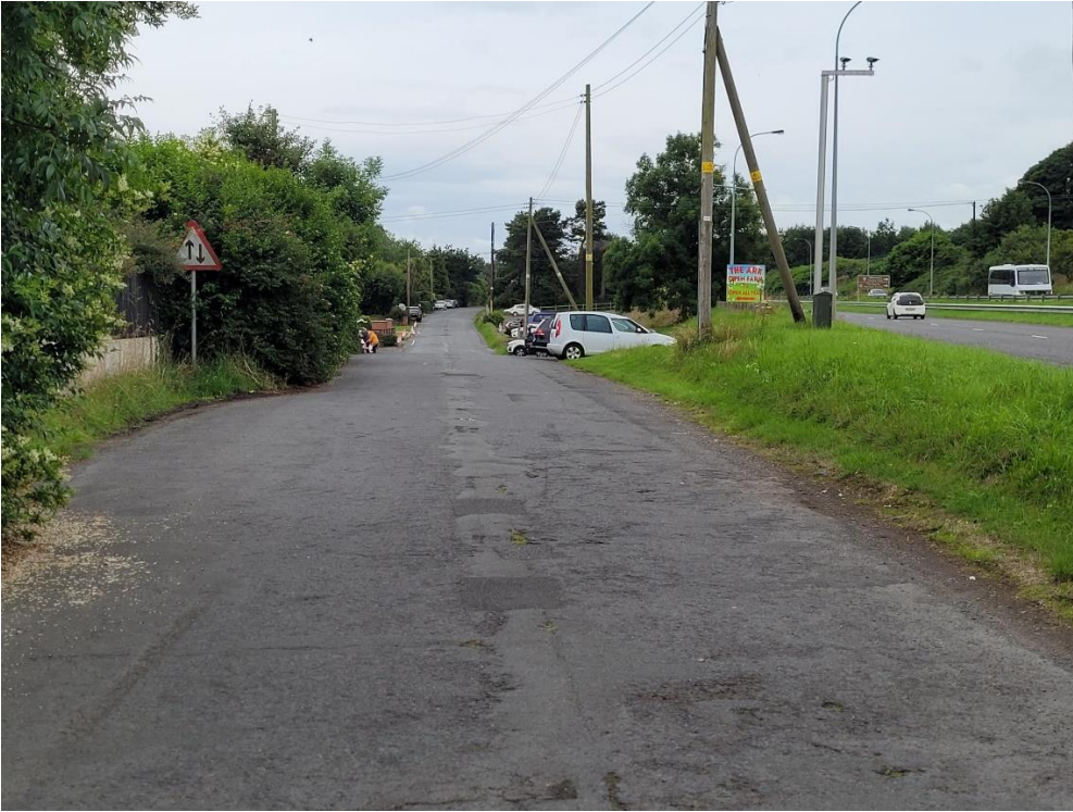
Photo 3 Looking back towards Bangor Road adjacent to dual carriageway
