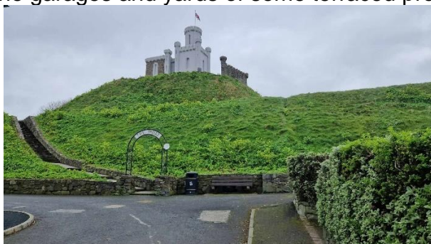
Figure 3: Moat Hill adjacent to rear of site
