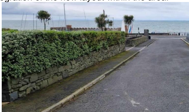
Figure 9: View of existing stone wall
