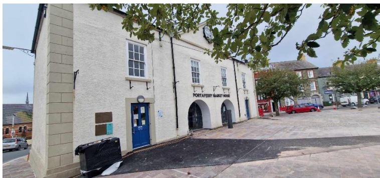
Front of building
