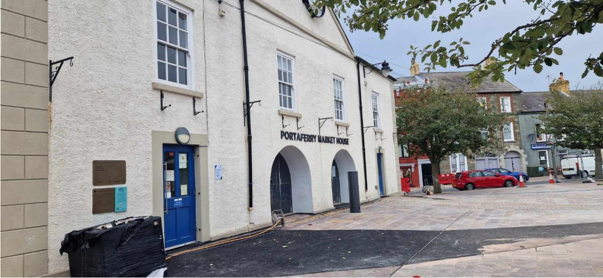
Front of application building
