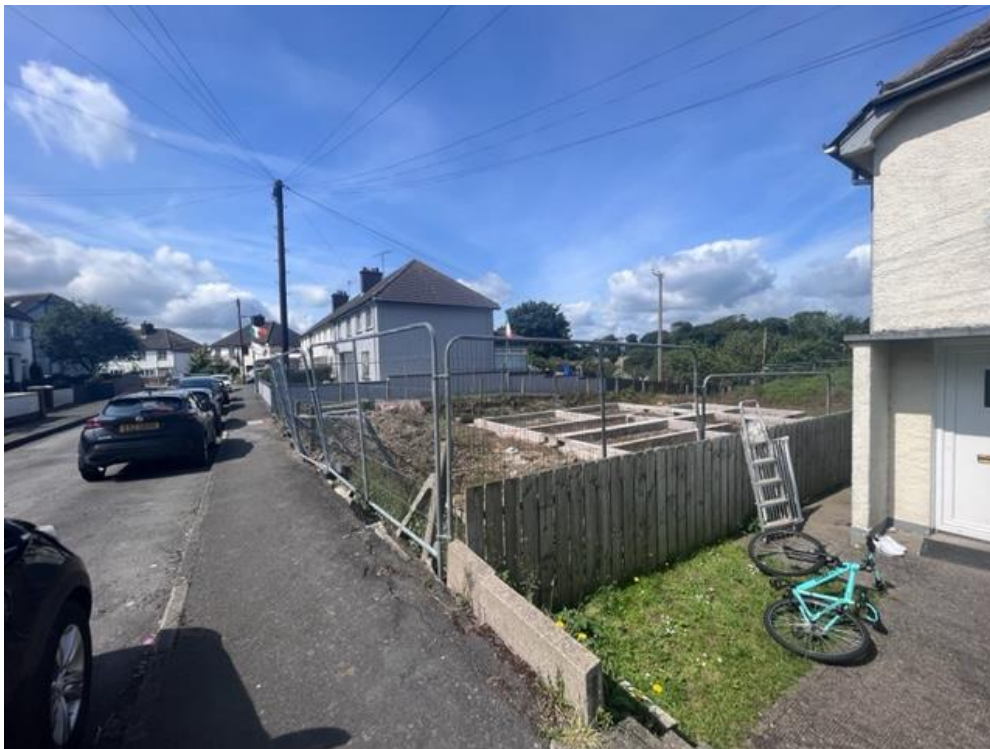
Foundations built for planning application ref. LA06/2017/0303/F
