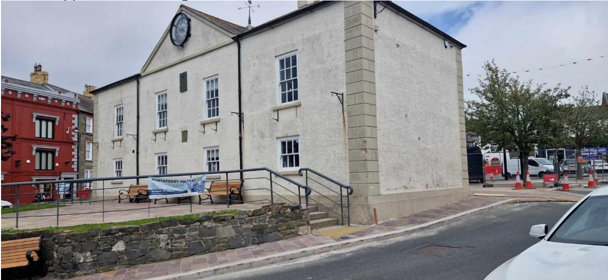
Looking to the southwest rear of building
