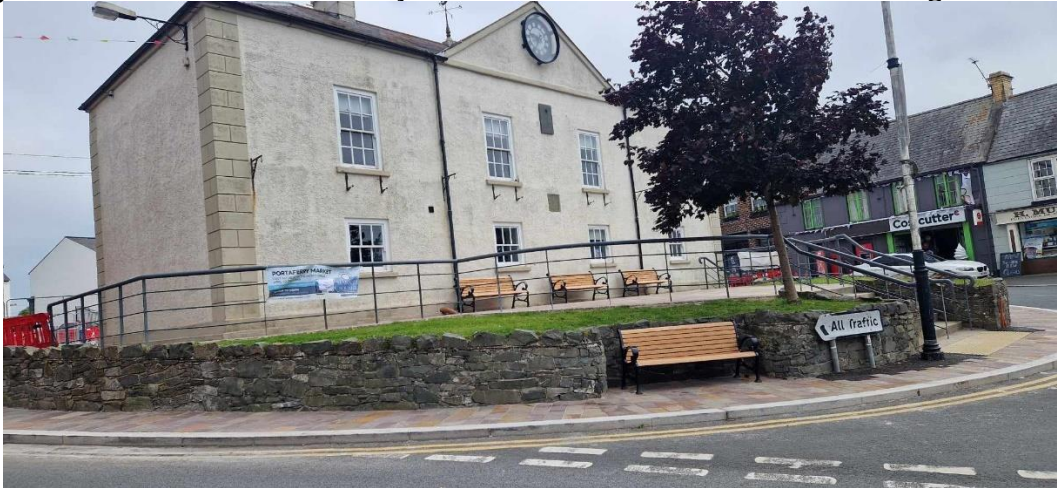
Rear of building with existing railing to the southwest – proposal shall match this
