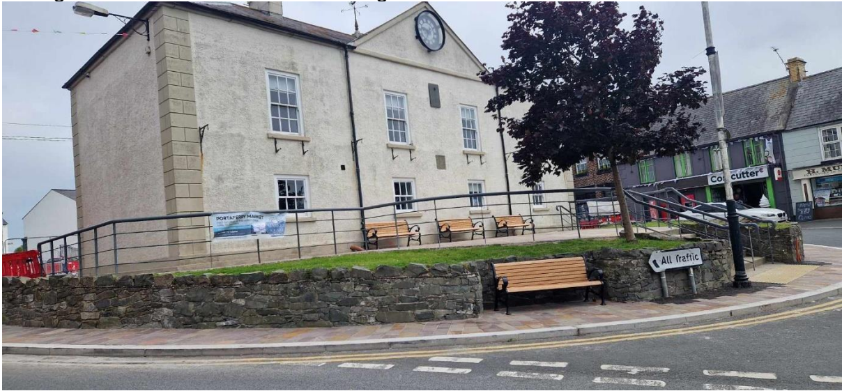
Looking to the southeast rear of building
