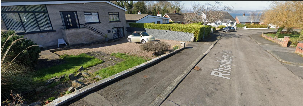
Figure 10: Front of Application Dwelling/Site
