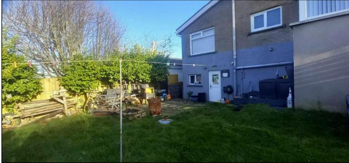
Figure 3: View from Application Sites Rear Garden Facing North
