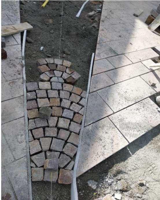
Intricate cobbling taking place in and around Market Square as the paving design begins to take shape
