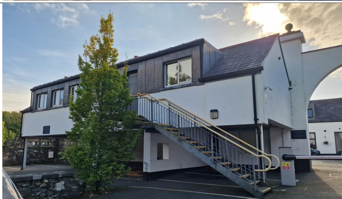
Existing Site Photographs
