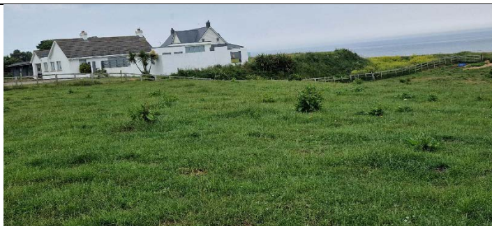
No. 38 Springvale Road to the north
