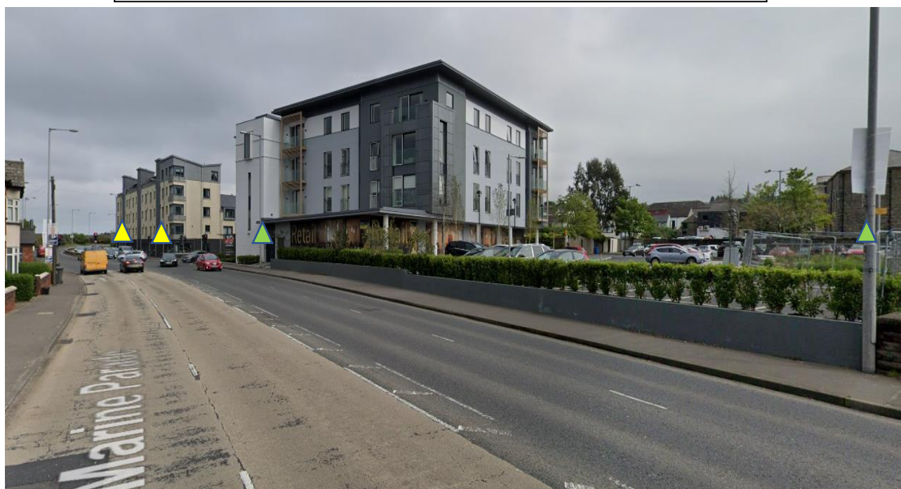
Figure 2.11 Holywood junction A2
