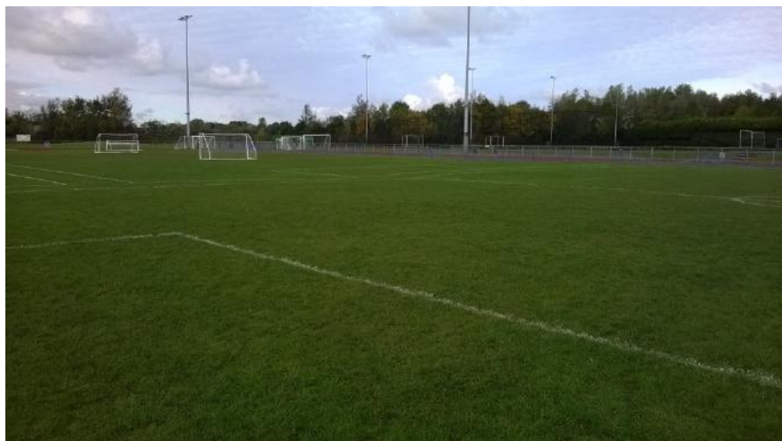
Photo 41 - Settlement in track infield
