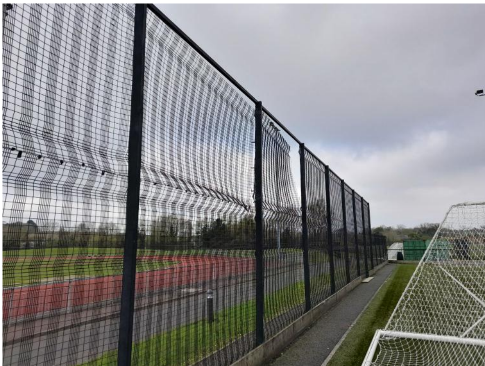
6 – Existing Fencing System
