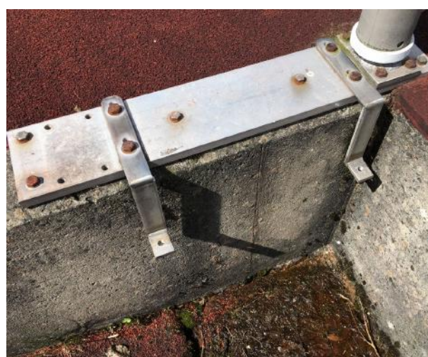
Figure 12 Pit surface and exposed edges
