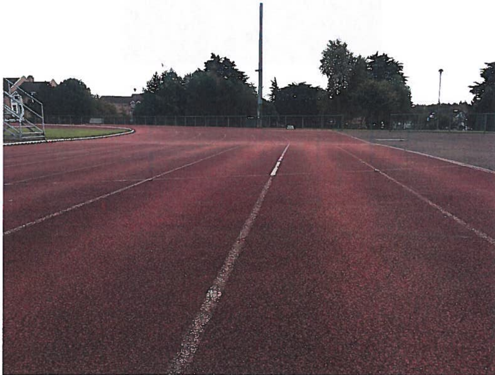
Area where kerbs, macadam and track have sunken creating a major dip in the track
