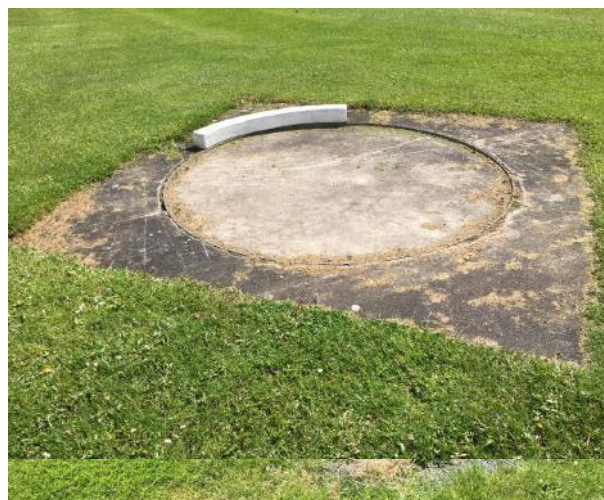
Figure 20 Shot 1 Natural grass infield landing area
