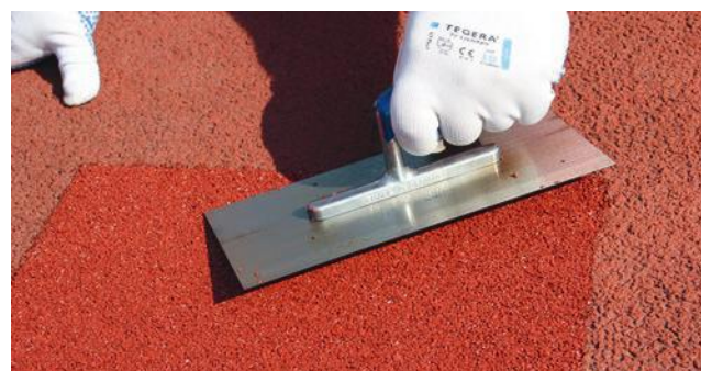
Repaired synthetic surface
