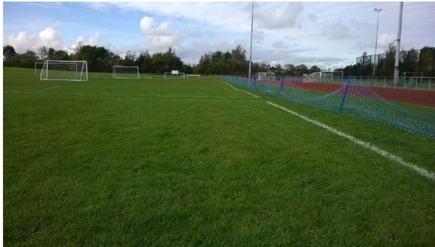
Photo 45 - Settlement in track infield
