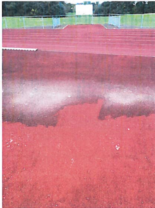
Area where track surface has been cleaned
