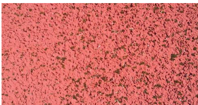
Bad example: Moss-covered synthetic surface
