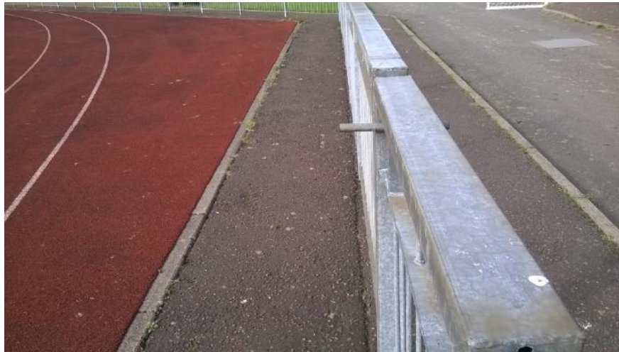
Photo 1 – Protruding latch at gate
