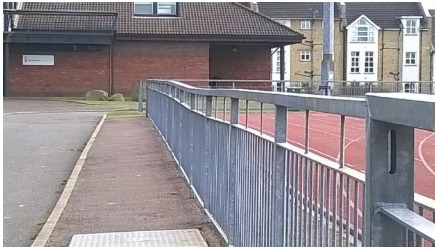
Photo 10 – Depression in spectator fencing at start of back straight.
