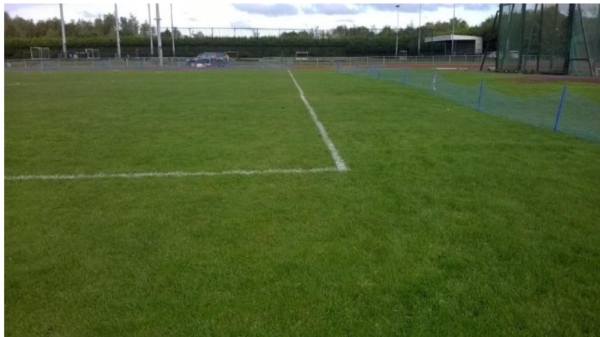
Photo 43 - Settlement in track infield
