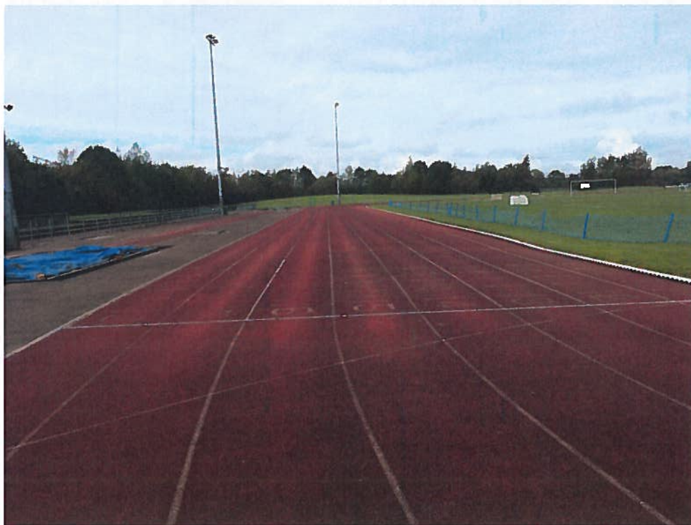
Wear of running lanes from use over time
