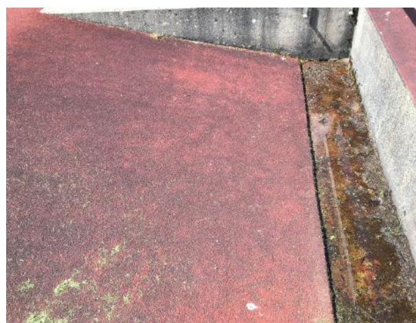
Figure 11 Cleanliness of pit
