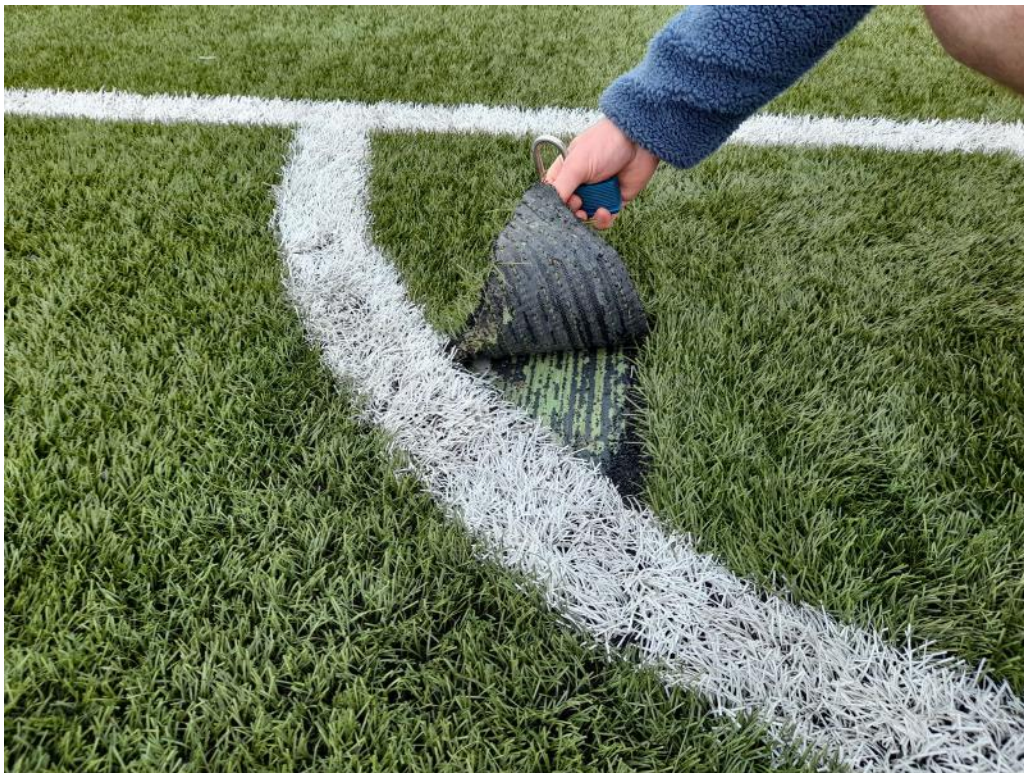
8 – Open Joint/ Seam
