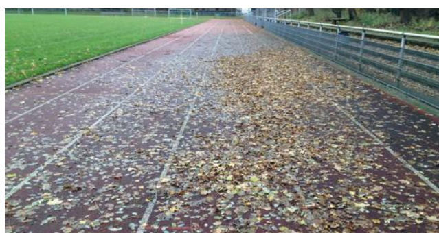
Bad example: Very dirty synthetic surface
