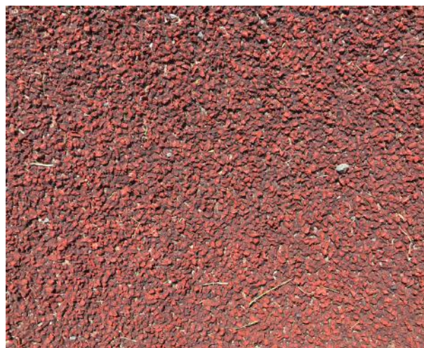
Figure 3 Typical track condition, high level dirt
