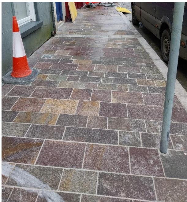
Works almost complete on the West footway
